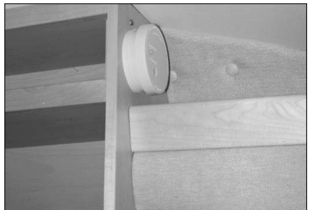
Picture F-P3: Smoke detector.
