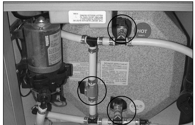
Picture G-P4: Winter mode valve positions.
