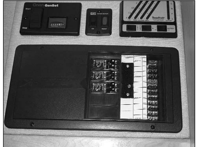
Picture E-P1: Monitor panel, water heater switch, 110/12V distribution panel and optional generator control switch.
